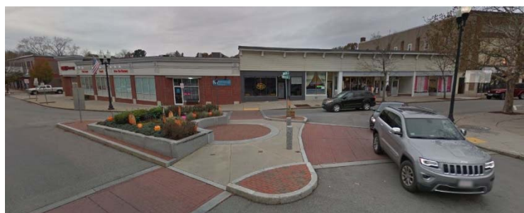
Nason St. at Main St. intersection, Looking west from Main St
