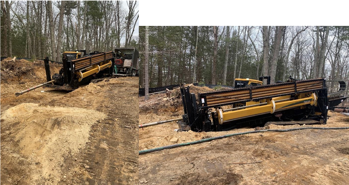
Photo – Horizontal Directional Drilling – Machine setup and drilling
