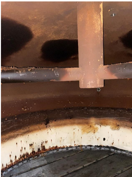
Filter 2 - internal distribution piping.
