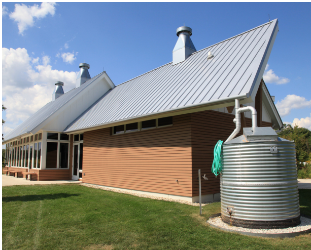
A cistern to capture roof runoff for irrigation.
