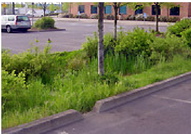
Above: A rain garden that infiltrates runoff.
